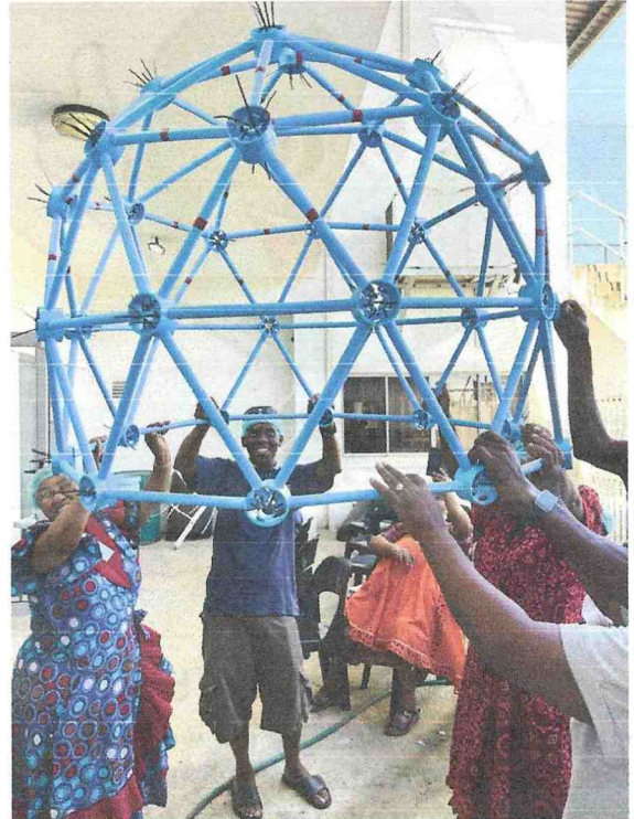
Holding up the completed mushroom silo dome frame
